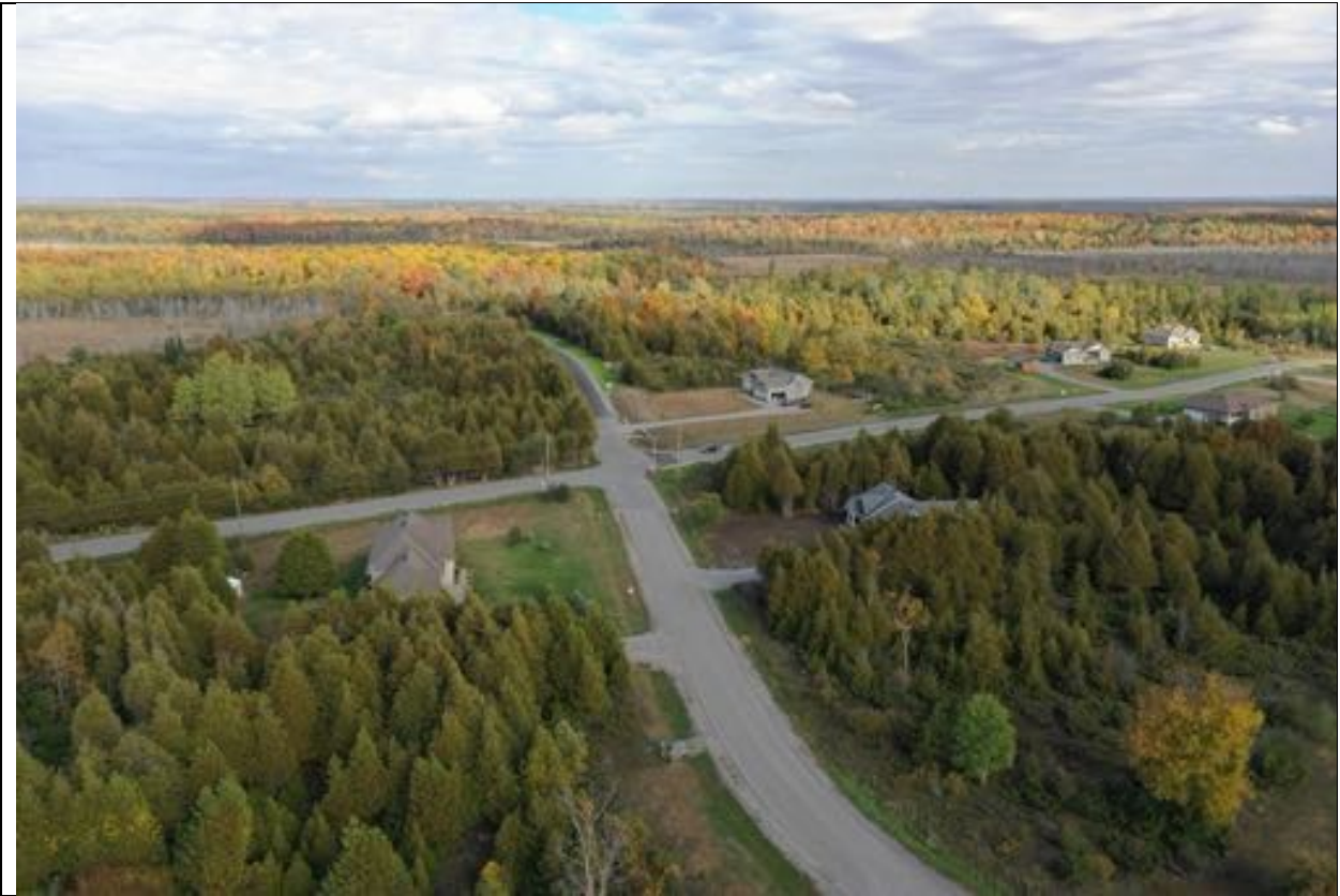
Phase 1 looking at Phase 3
