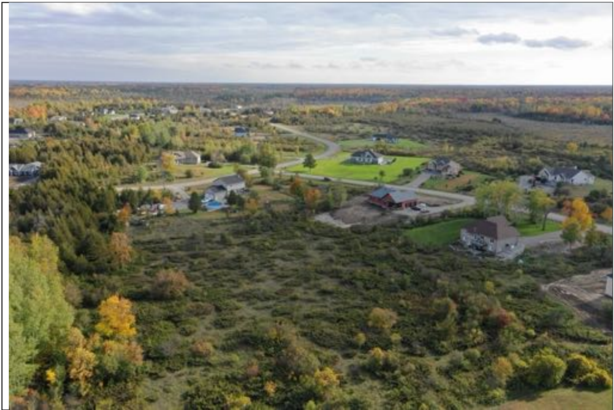
Phase 1 looking at Phase 2
